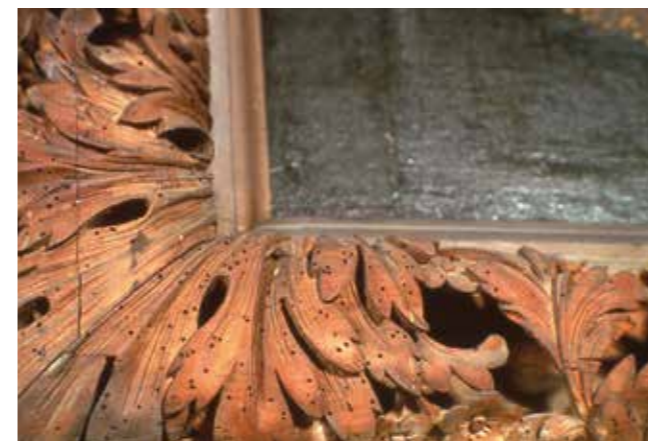
Woodworm damage (National Trust Images)
